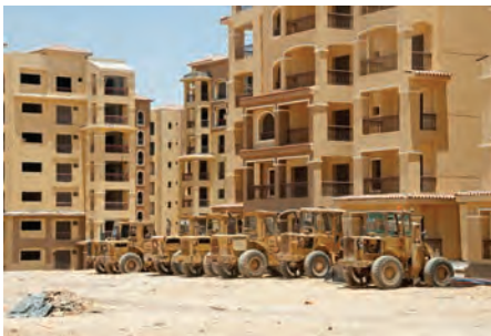
Construction machinery parked in front of residential buildings in New Cairo next to the Cairo Suez Road
