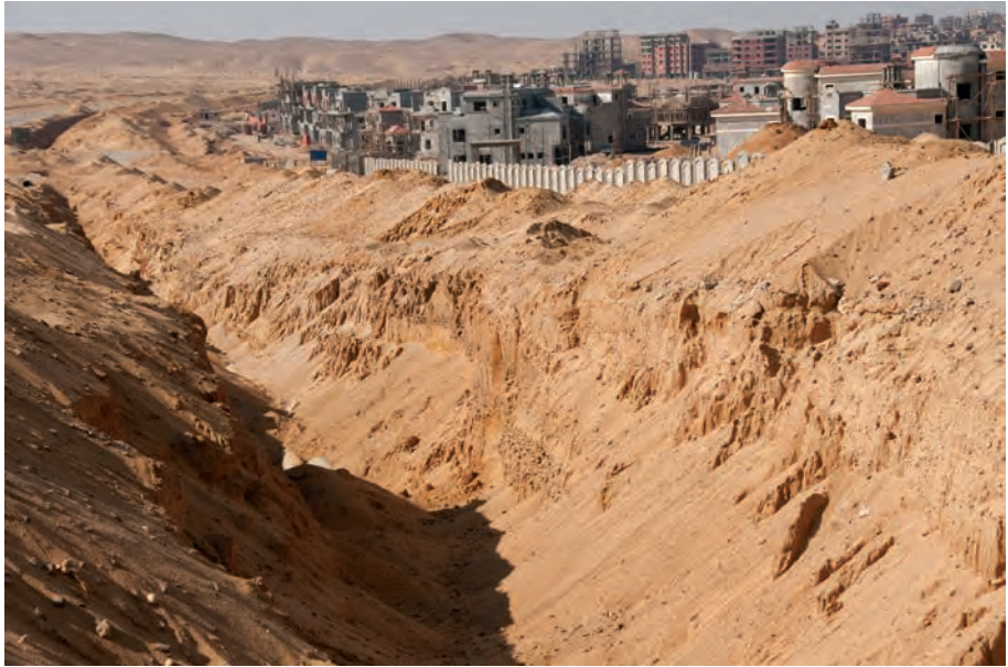
A view towards New Cairo to the South not far from the American university. Gated communities are under construction. In the foreground work is taking place to install the city's infrastructure.
