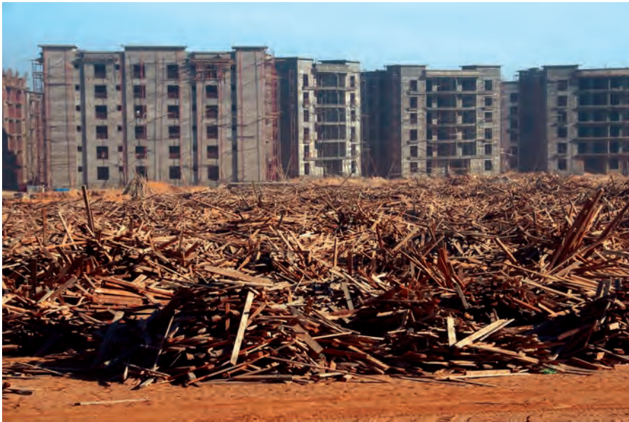
Apartment buildings under construction with removed wooden scaffolding standing on the ground in the foreground.
