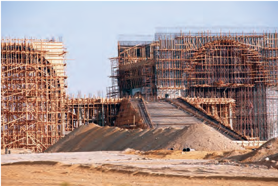
This image corresponds to an unfinished entrance of one of the largest mix used complexes in New Cairo, which will have shopping centers, corporate buildings, villas, golf courses, and apartment blocks.
