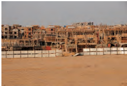
Frontal view of a gated community under construction
