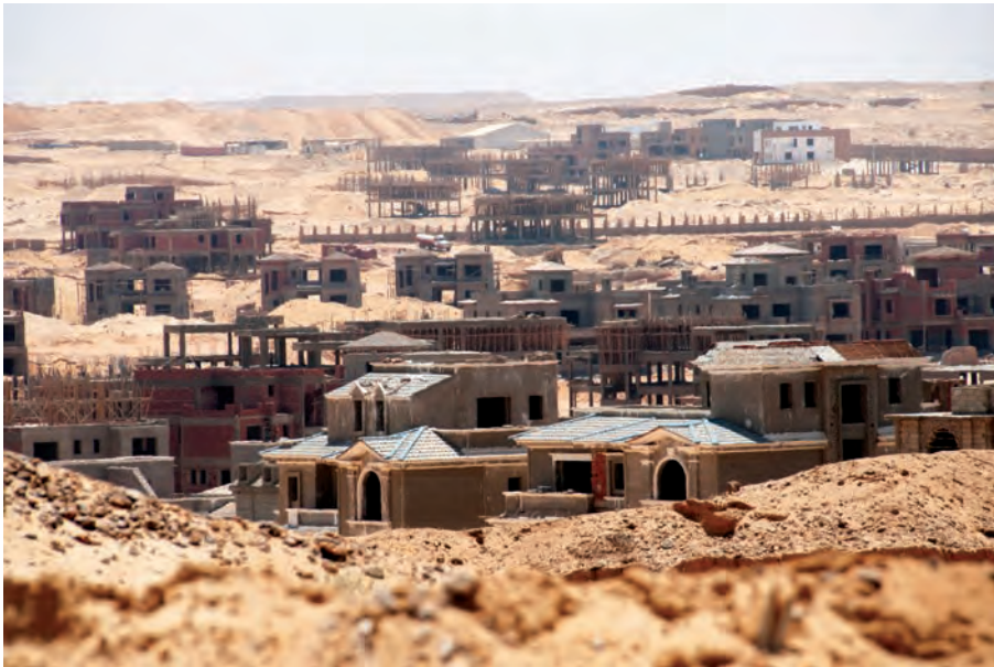
A gated community in construction seen from a hill
