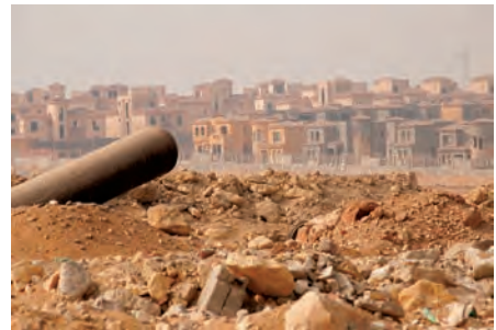
A view of an almost finished gated community with a concrete pipe on the left margin pointing at it.
