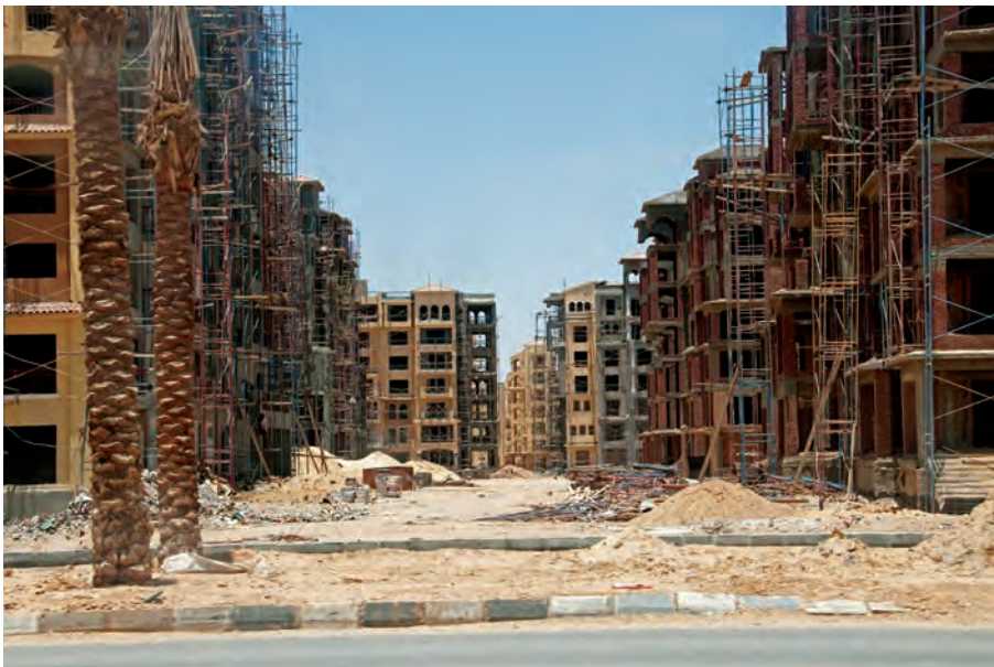
Apartments under construction in New Cairo. Driving along the Suez Road these structures can be seen occupying a vast territory of land.
