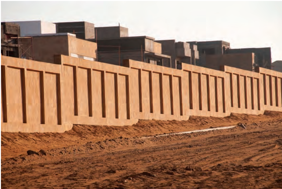
Security wall surrounding the perimeter of a gated community
