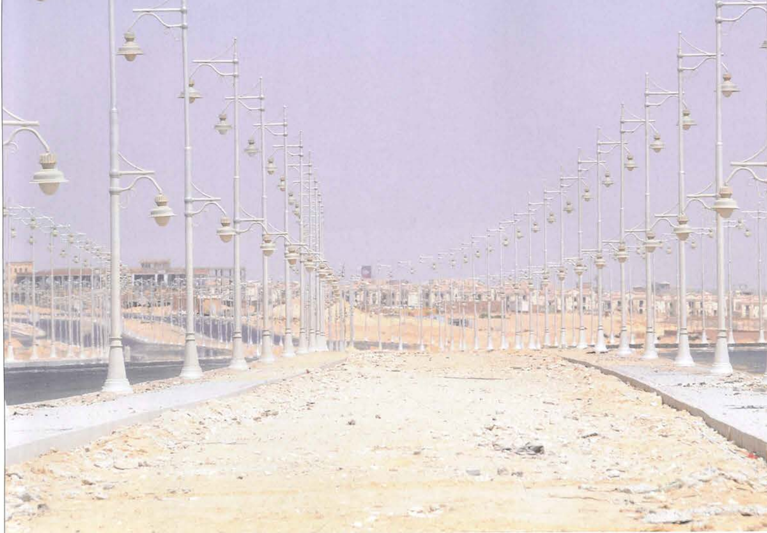
Corridor of lamposts on Moubarak Axis Road in New Cairo, which links the eastern part of New Cairo with its city centre. At this stage this major artery connects built areas to incomplete ones, or the desert
